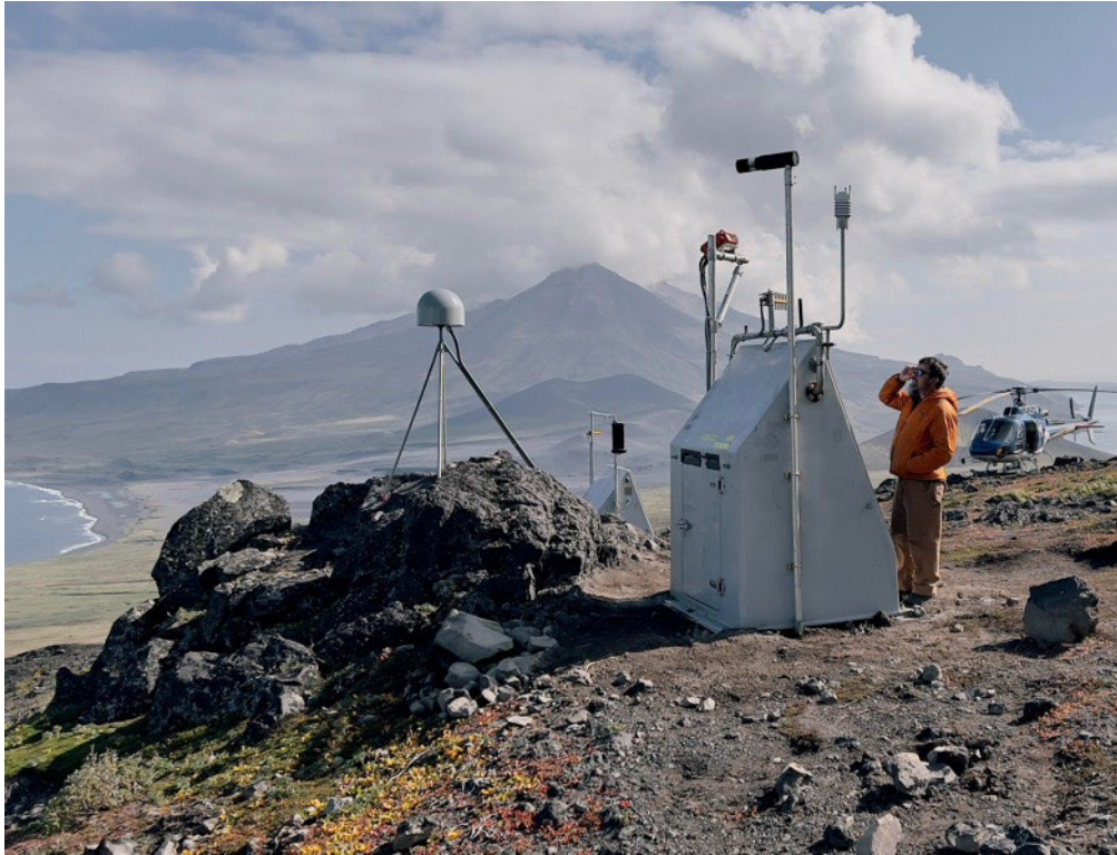
Hut-1 = Seismometer, GNSS, Magnetometer, Wind Generator
