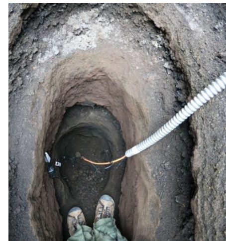
Soil probe installation Tarsilo Girona
