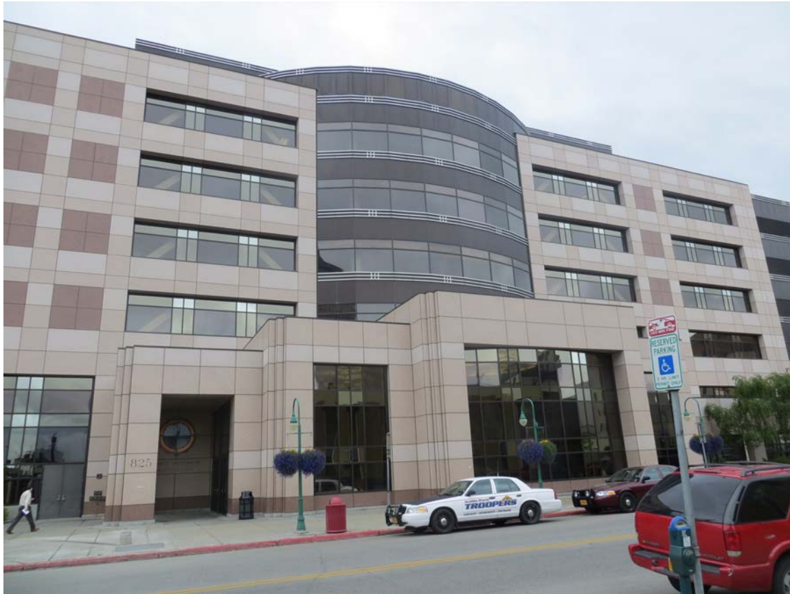
Figure 1.4. Nesbitt Courthouse. Note eccentric bracing in windows.
