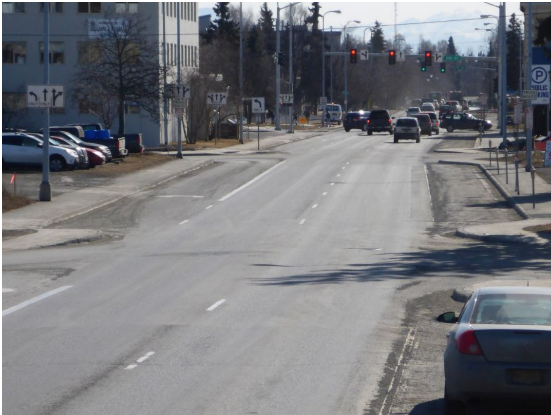
Figure 1.5. View looking south down L Street from a just south of 6th Avenue, Anchorage, Alaska. The two subtle but distinct kinks in the centerline, as it is traced from lower left toward the upper right, represent the re-alignment of L Street where it crossed the main scarp at the head of the L Street Slide (from Thoms et al. (2014).
