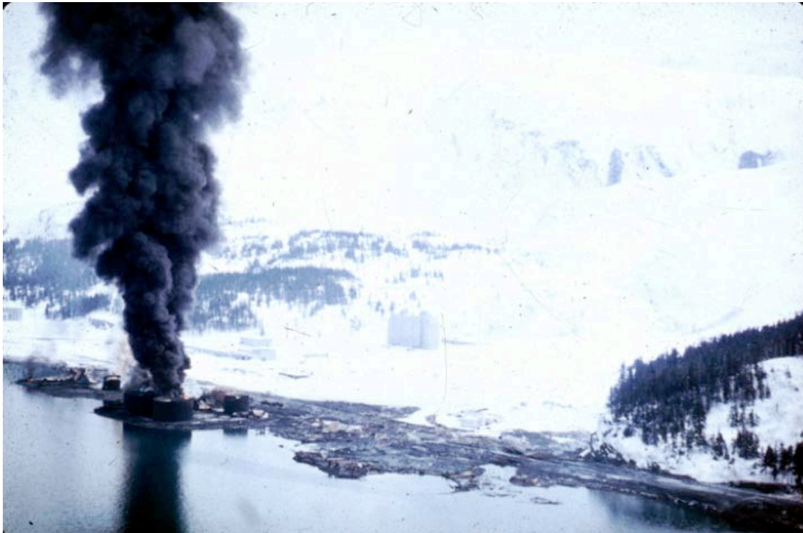
Figure 5.1. Alaska Earthquake March 27, 1964. The dock area, a tank farm, and railroad facilities at Whittier were severely damaged by surge-waves developed by underwater landslides in Passage Canal. The waves inundated the area of darkened ground, where the snow was soiled or removed by the waves (USGS).
