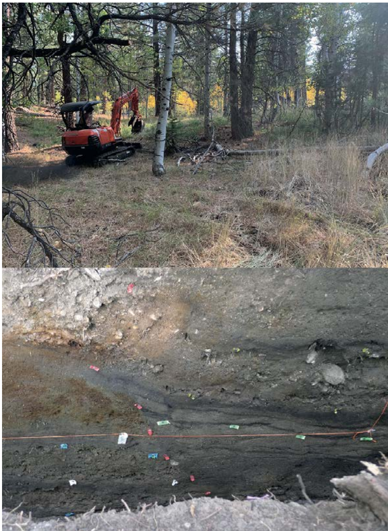
Figure 6. Upper: Photo of excavator at the toe of the fault scarp. Lower: east wall of the trench showing sharp juxtaposition of fluvial units across an apparently dipping fault.
