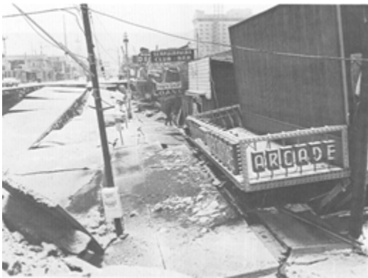
Figure 1. The head of the Fourth Avenue landslide induced by the 1964 Great Alaska Earthquake (Hansen 1971).
