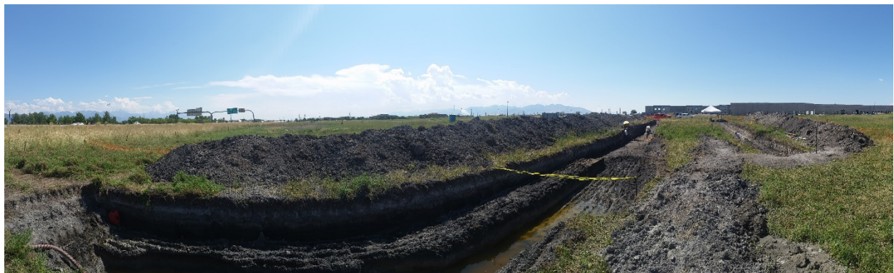
Figure 6. Panoramic photo of Airport East site, looking southwest into South trench. North trench visible on right.
