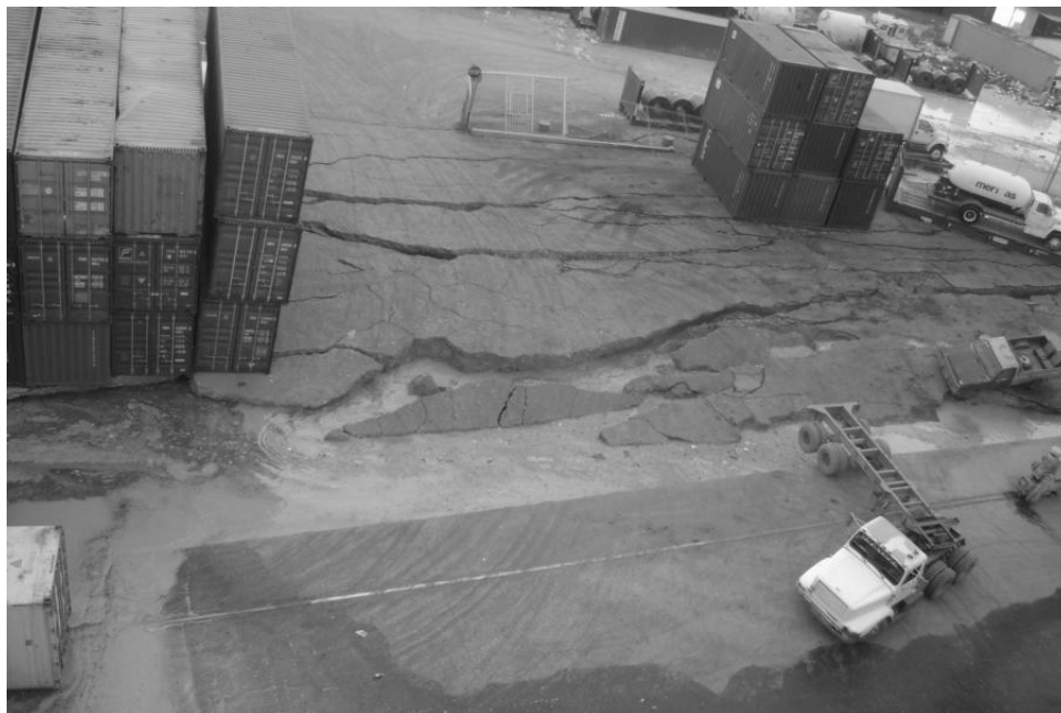
Figure 2-7: Lateral spreading at the port in Port-au-Prince, Haiti following the 2010 earthquake (courtesy of EERI)
