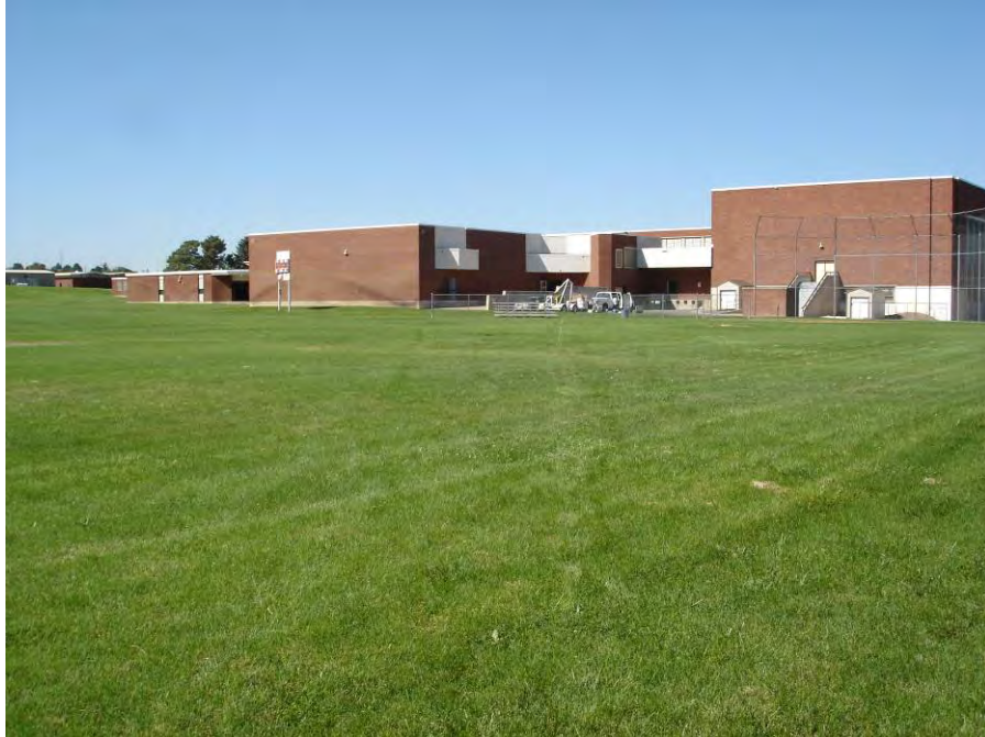
Fig. 2.74 Photograph of SASW testing at South Ogden Junior High School (SOJ), Weber County, Utah.
